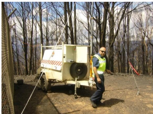
Radio Tech from Morwell, Tony Desira lashing the mast and trailer down to ensure no more wind damage occurs.
