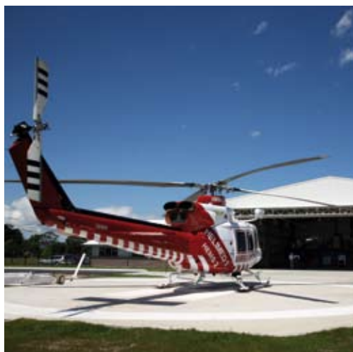
The new facilities at the La Trobe Valley for the HEMS-2 helicopter, which is operated by MAS.
