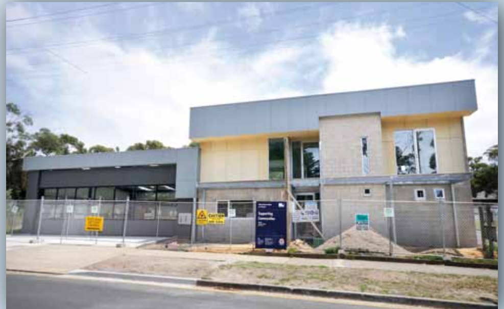
The new branch under construction.
